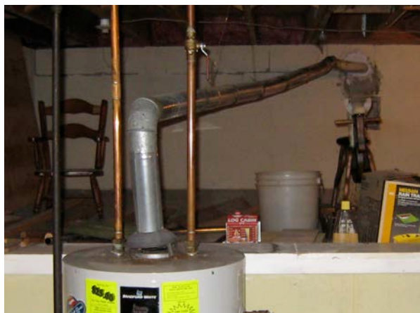
Photo 3. Long Low-Slope Flue Pipe
