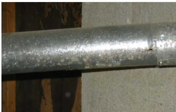
Photo 2. Rust on Flue Pipe
