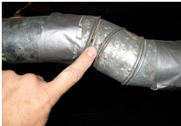
Photo 4. Metal Flue with Holes, Tape
