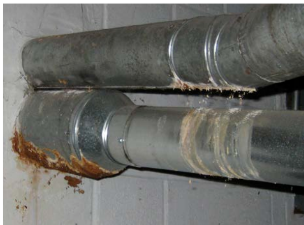
Photo 1. Signs of Condensation
