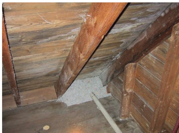
Photo 2. Plugs in Floor – Cellulose
