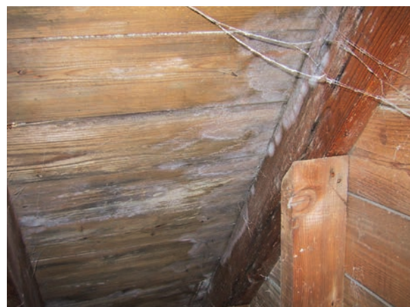
Photo 3. Attic Mold Growth
