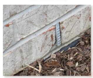
Photo 2. Brick Veneer Flashing and Weep
