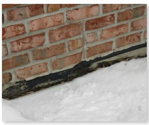
Photo 1. Brick Veneer Flashing
