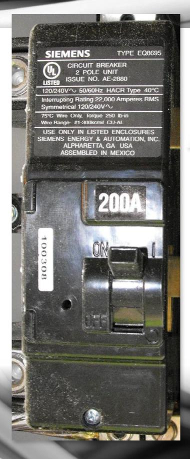
Because most electrical service panels are not installed by homeowners or "Uncle Harry," it is rare to find service equipment without a means of disconnect. There are a couple of ways where it might appear to be missing, but is in fact there after all. I want to keep this post simple enough that most readers can understand what I am talking about.
