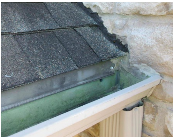
Photo 2. Adhered Stone - No Kickout Flashing
