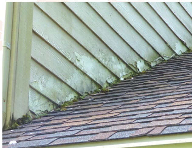
Photo 1. Siding damage, no clearance.
