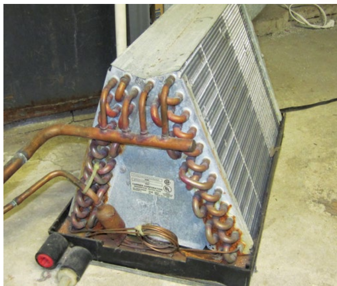
Photo. Air Conditioner A Coil
