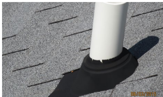
Photo 1. Cracked vinyl flashing
