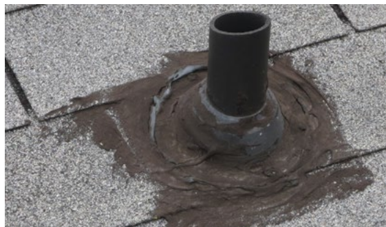
Photo 2. Tar-coated flashing
