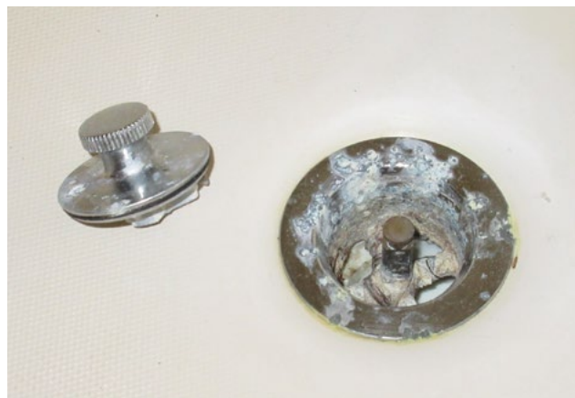
Photo 3. Excessive corrosion.
