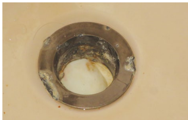
Photo 2. Surface corrosion.
