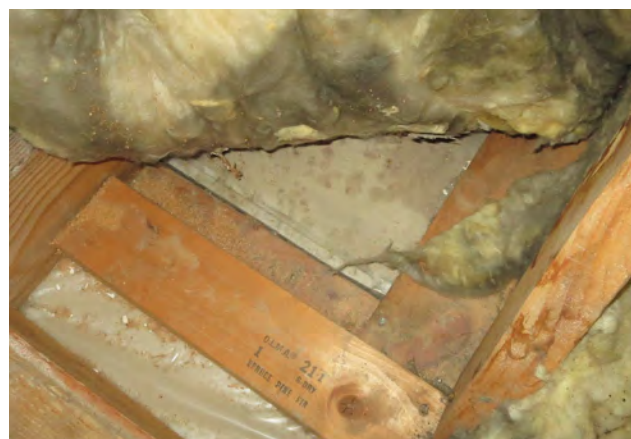
Photo 2. Wood Shrinks and Air Leaks.
