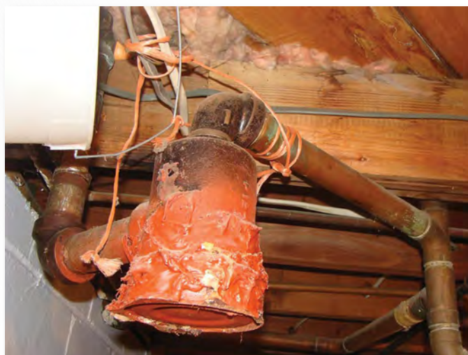
Photo 16. Hack drum trap repairs.
