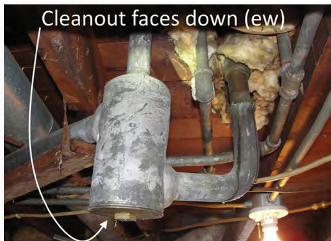
Photo 4. Drum trap with cleanout facing down.
