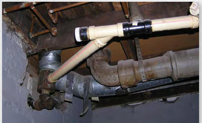
Photo 11. Mixed drains with drum trap.
