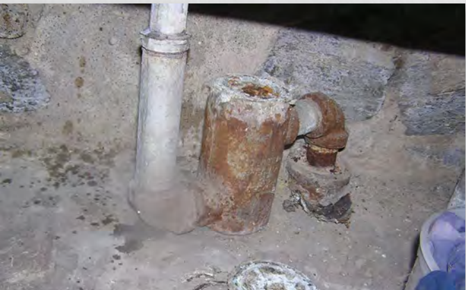
Photo 9. Corroded cap at drum trap.
