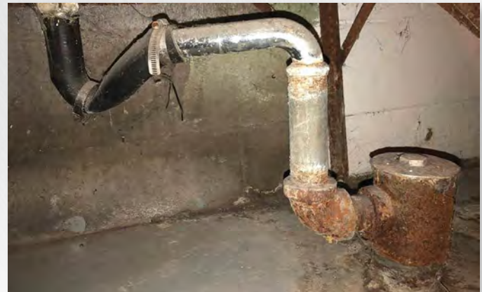
Photo 12. Radiator hose trap.
