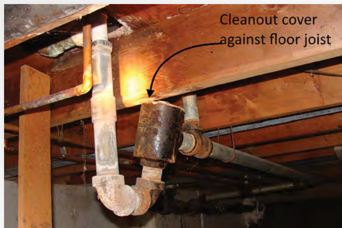
Photo 3. Drum trap with blocked cleanout
