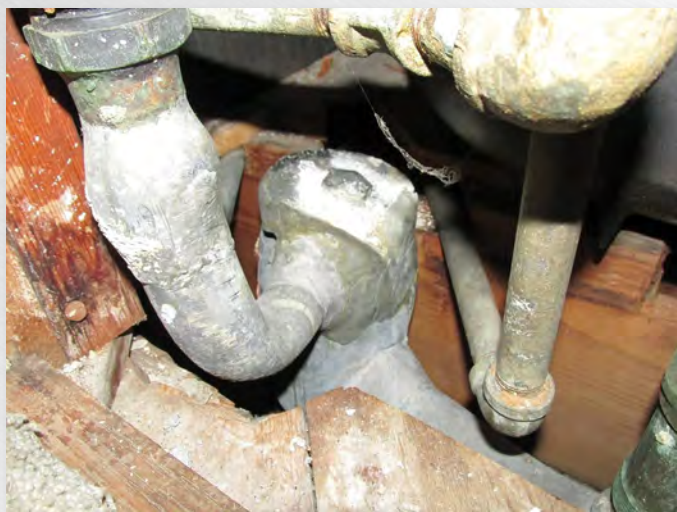
Photo 6. Lead drum trap with makeshift repairs.
