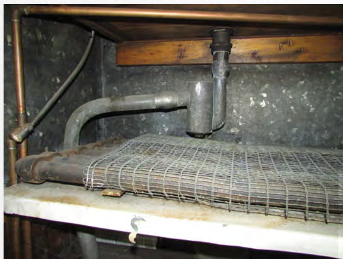
Photo 14. Drum trap in butler's pantry.
