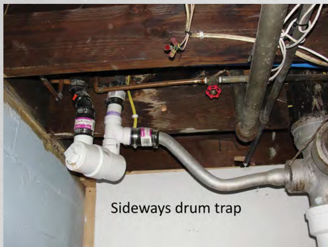
Photo 5. Sideways drum trap.
