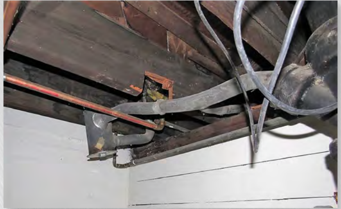
Photo 10. Notch in floor joist.
