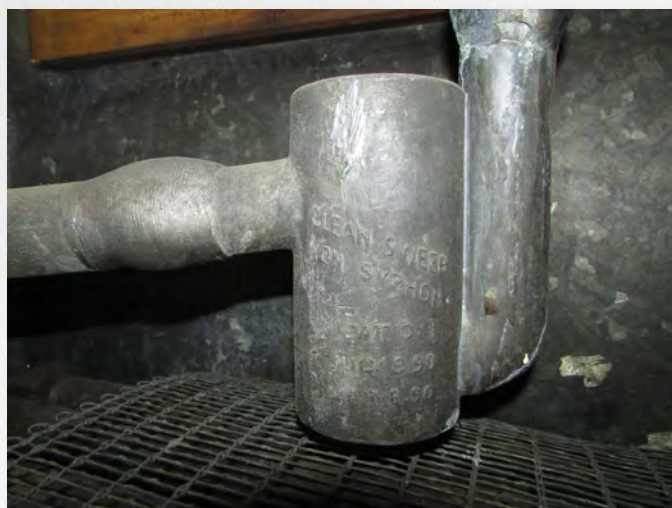
Photo 13. Drum trap in butler's pantry.
