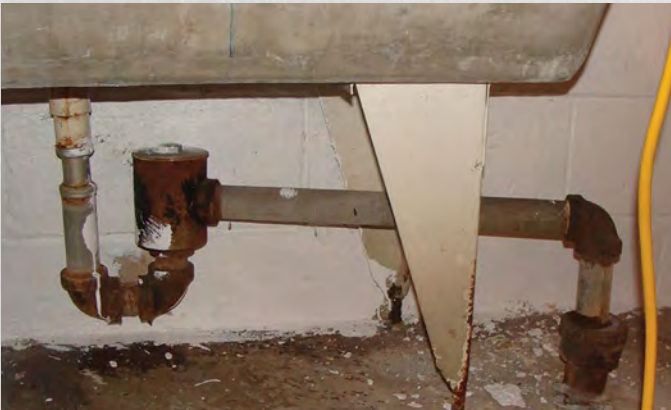
Photo 8. Drum trap at laundry sink.
