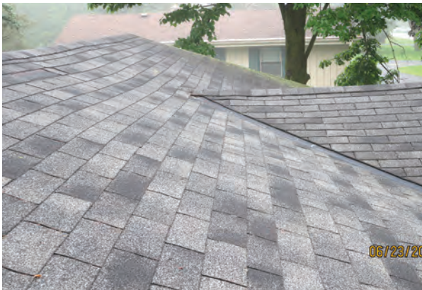
Photo 1. Visible roof sag.
