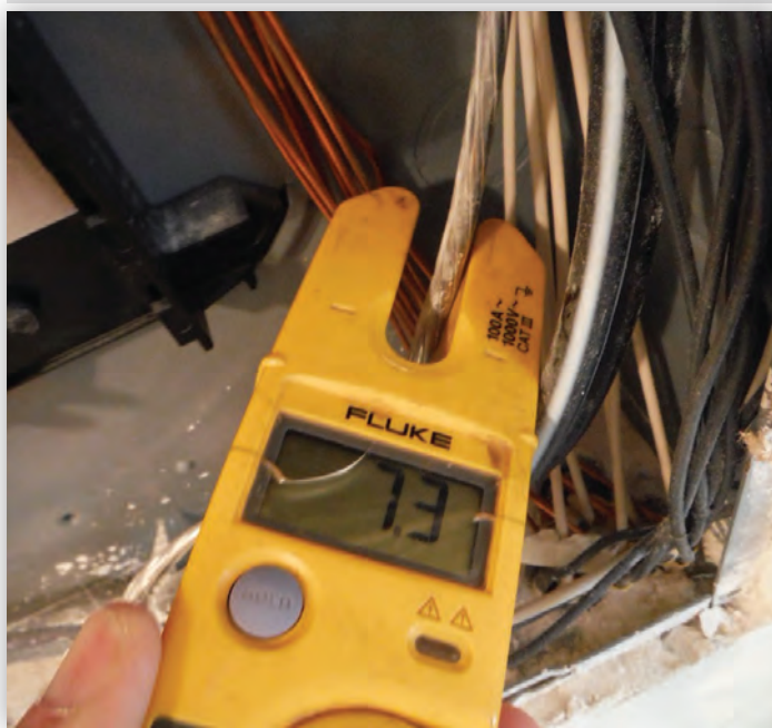
Dangerous current (7.3 amps) on equipment grounding conductor from improper load side neutral bonding.
