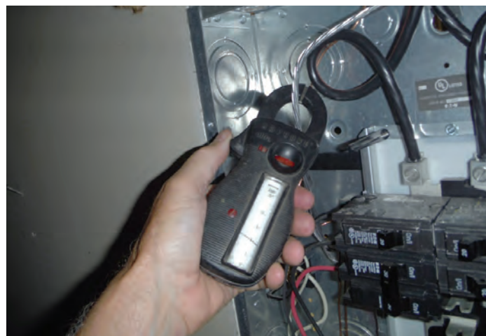
6 amps on EGC (neutral improperly bonded).
