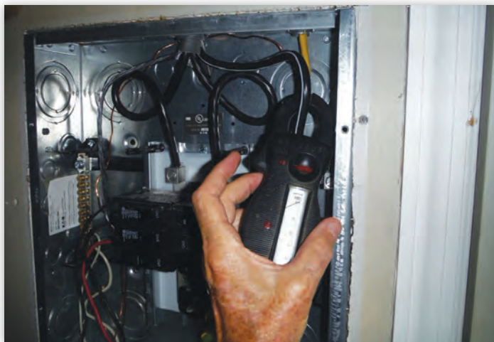
Properly wired subpanel (neutral, not bonded). All 15.5 amps are on the neutral feeder.
