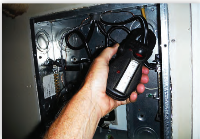
Neutral improperly bonded; 9.5 amps on neutral feeder.
