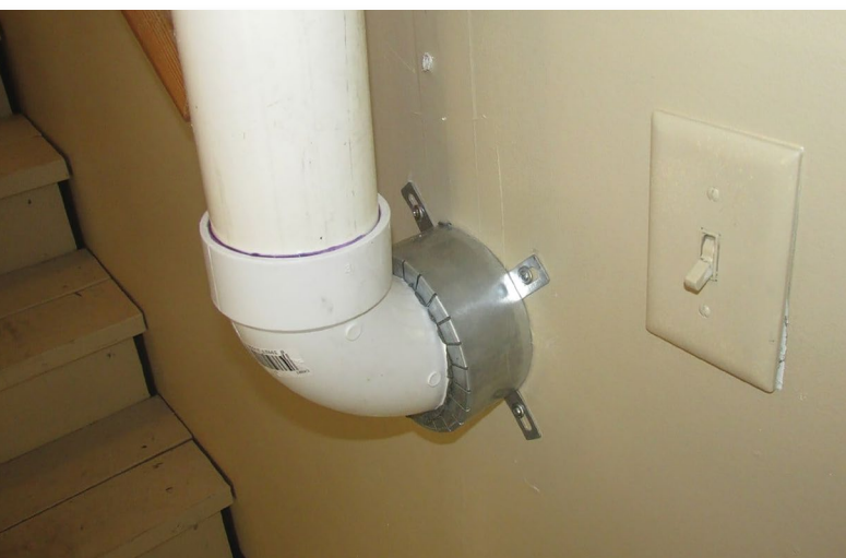
Photo 1. Firestop collar for a radon mitigation system
