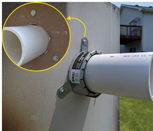
Photo 9. Firestop collar, proper installation.
