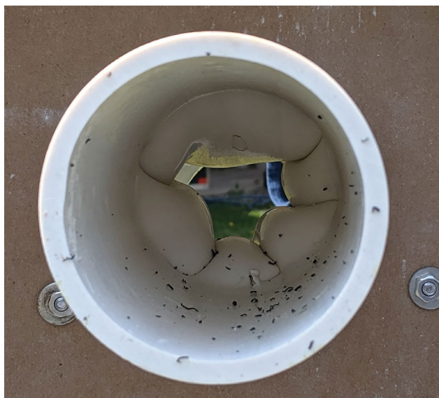
Photo 10. Firestop collar, proper installation.
