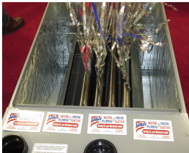
Photo 2. Condensing furnace air movement.
