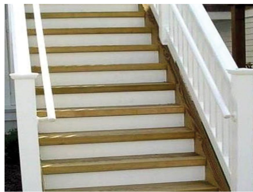
Stairs that are completely closed and do not meet the requirement to allow the flood waters to pass through them.
