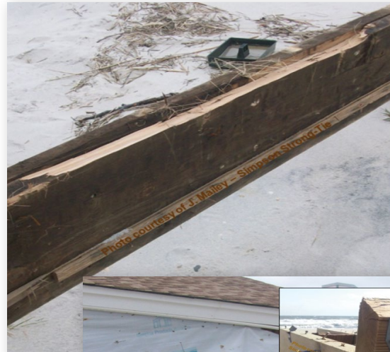
A beam in a home that was rebuilt after being destroyed by a flood. The joists are resting on the beam and the beam is sitting on the pier. Nothing is tying the framing to the foundation. Unfortunately, this home will be subject to floating away in the next flood.
