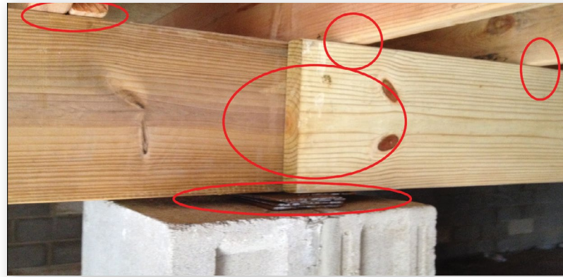
A beam in a home that was rebuilt after being destroyed by a flood. The joists are resting on the beam and the beam is sitting on the pier. Nothing is tying the framing to the foundation. Unfortunately, this home will be subject to floating away in the next flood.
