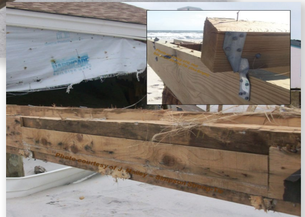
Note the wood failure or tearing perpendicular to grain because the connector fasteners were too close to the edge of the wood.
