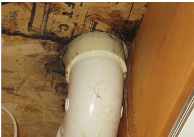
Photo 4. Water Damage Below Toilet.
