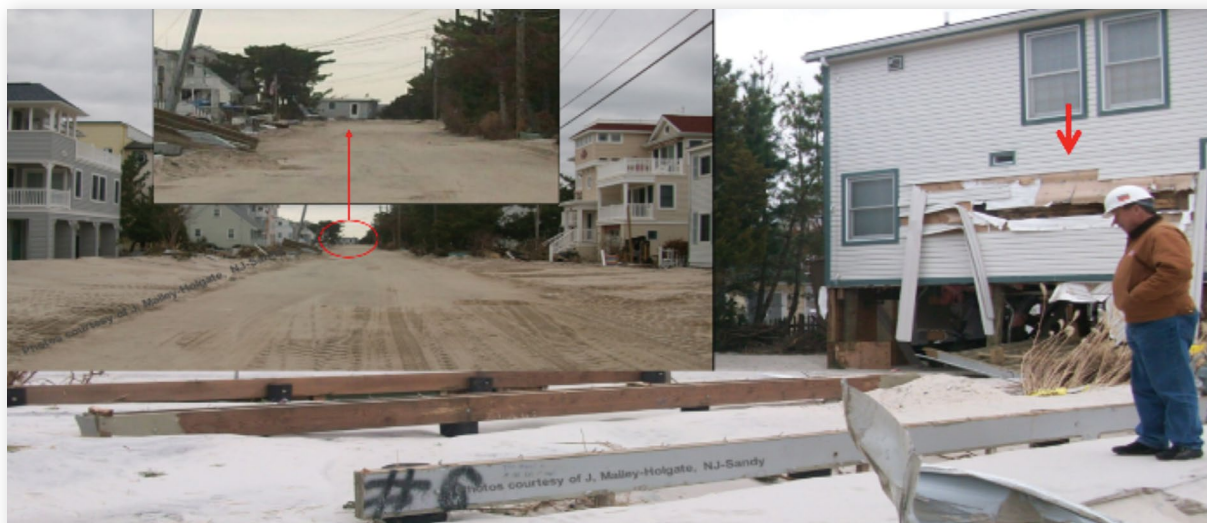
This home lifted off of the foundation, knocked into the house next door, and floated down the street about 600 yards and sits in the bay at the end of the road.
