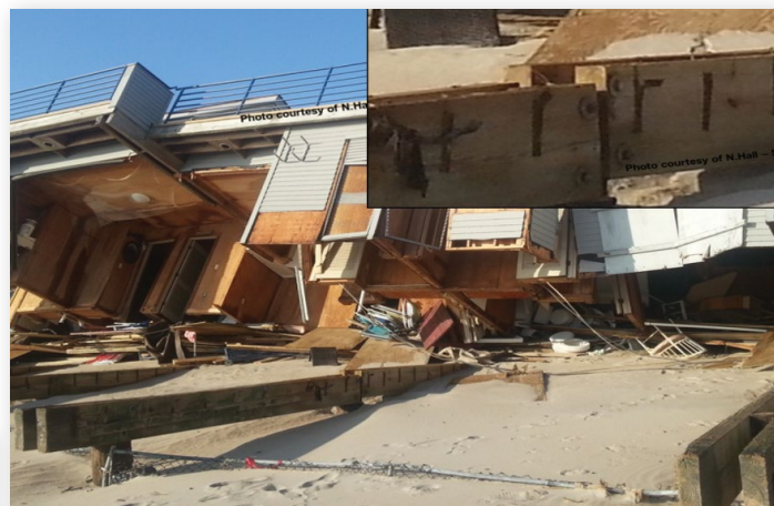
The straps connecting the beams to the joists failed during a flood event due to inadequate corrosion protection of the metal.
