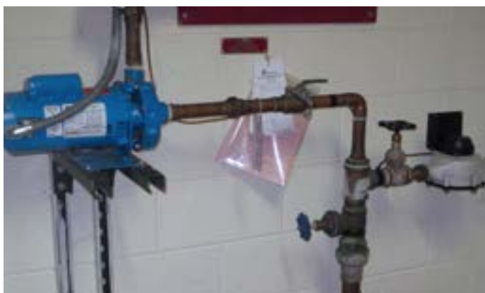
Photo 2. Water main booster pump.
