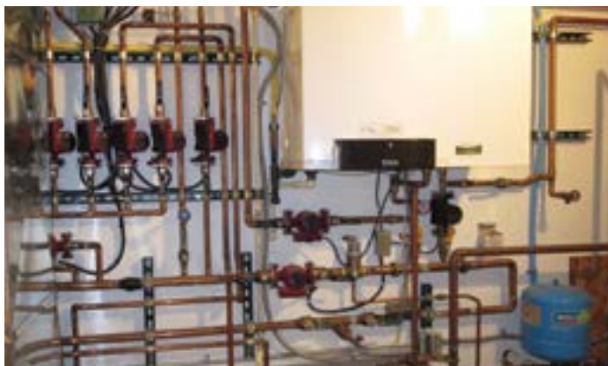
Photo 1. Heating system pumps.
