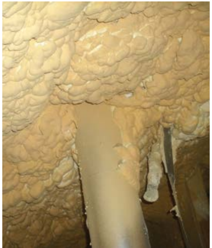
Photo 1. Can you tell if this spray foam insulation is installed according to the test conditions? The Word can't.
