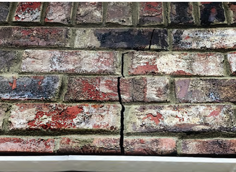
Photo 3. Shear crack.
