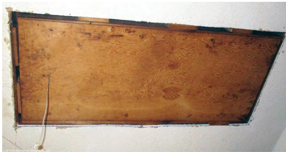
Photo 8. Pull-down stairs are almost always wrong in a garage.
