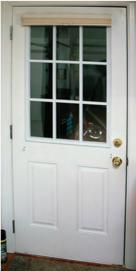
Photo 6. Glass in a door to the garage is a fire separation defect, but The Word doesn't lose any sleep about this one in his house.
