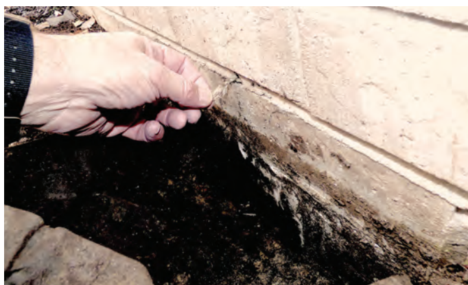
Photo 4. Weep high on the brick.
