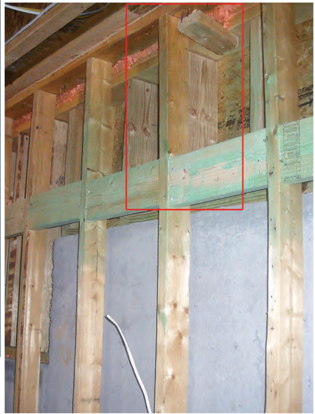
Photo 3. Fireblock double walls every 10 feet both, as shown in the red box, and also along the foundation.
