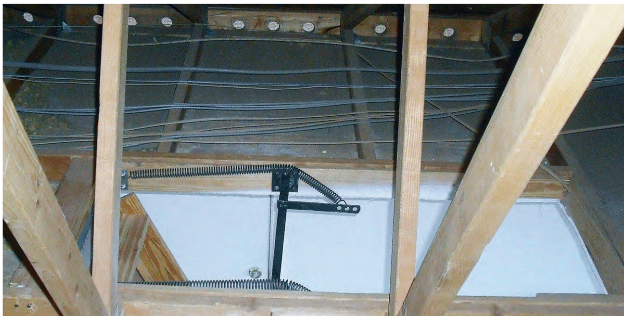
Photo 9. Couldn't they have installed it between the chords and avoided an expensive repair?
