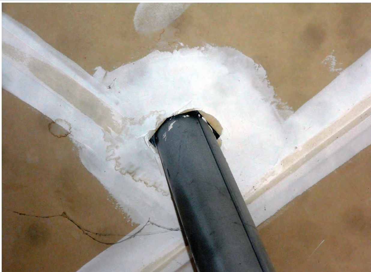
Photo 10. There should be a metal escutcheon where this water heater vent penetrates the garage ceiling.
