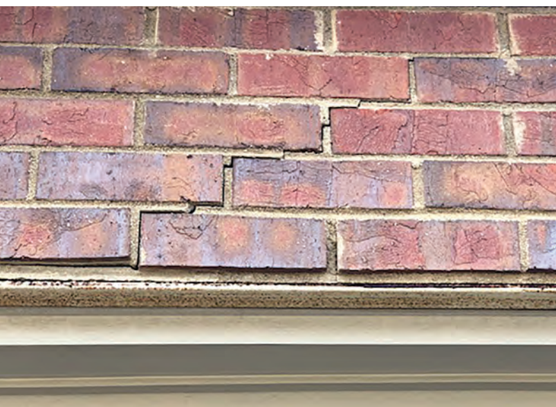
Photo 4. Stairstep crack.
