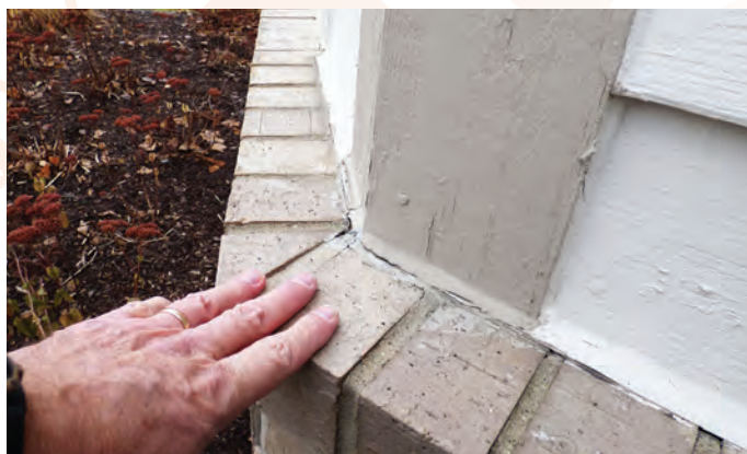
Photo 3. Cap with no slope or flashing.
