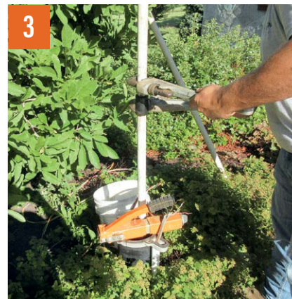
Photo 1: Pulling the submersible pipe and pump. 2: Pipe, pitless adapter, orange clamp. 3: Removing section of pipe. 4: Pipe, old pump, and casing.
