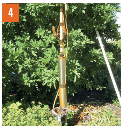
Photo 1: Pulling the submersible pipe and pump. 2: Pipe, pitless adapter, orange clamp. 3: Removing section of pipe. 4: Pipe, old pump, and casing.
