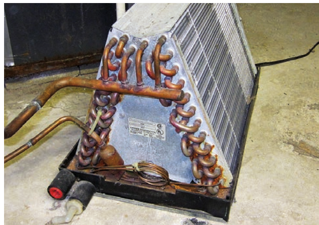
Photo 3: Air Conditioning A Coil
