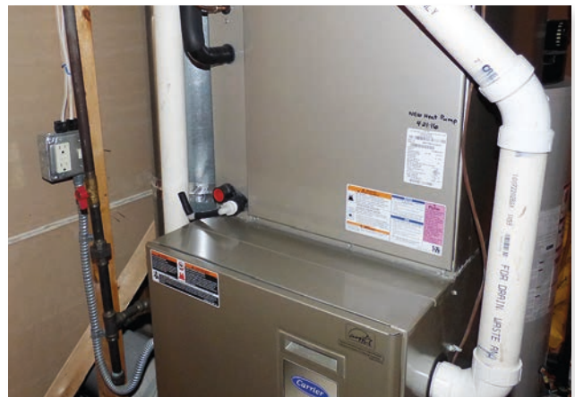
Photo 1: AC Coil Connections at Furnace
