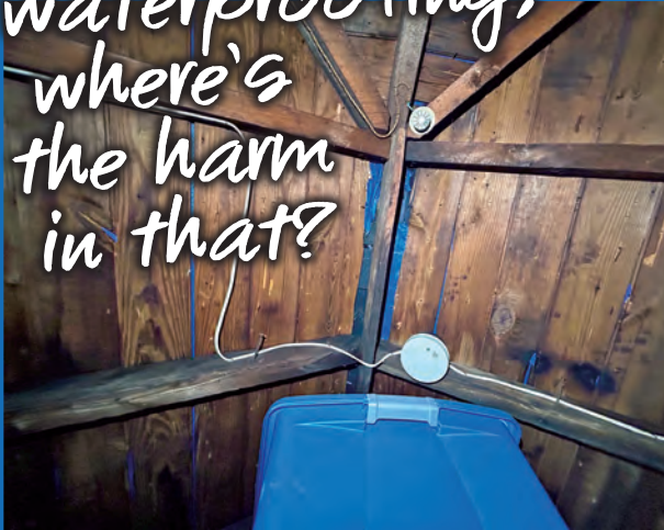
Michael Sutton | Ocean Home Inspections Oakhurst, NJ
