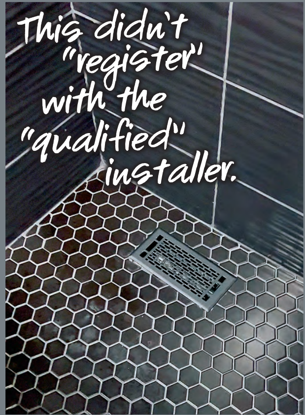
Nick Boese | Iron Gate Inspection Services Indianapolis, IN
