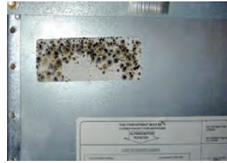
Mold growth on the label in a blower cabinet
