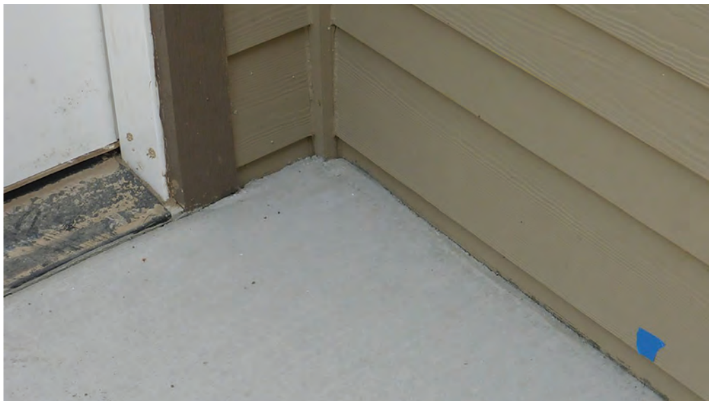
Photo 3. Concrete Installed in siding contact—a common installation error that is typically not cost-effective to correct until needed.
