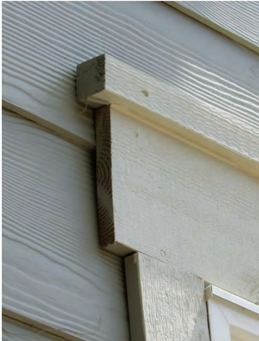
Photo 1. Cap-over trim detail on new construction.
