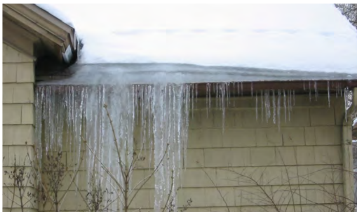
Photo 2. Ice dam east gutter
