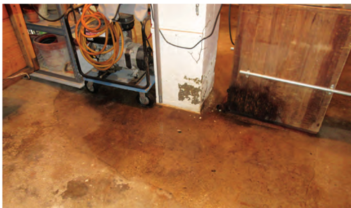
Photo 2. Leaks into center of garage
