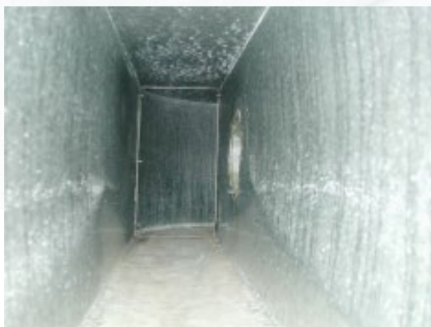
Photo 3. Winter condensation in attic air-conditioning supply duct. May Indoor Air Investigations LLC
