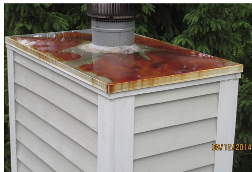
Photo 1. Metal cap with rust and drainage problems
