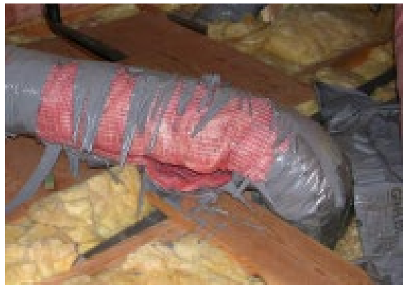
Photo 2. Degraded flexible duct in attic. May Indoor Air Investigations LLC
