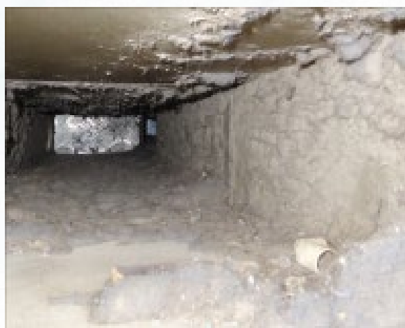
Photo 4. Filthy return duct. May Indoor Air Investigations LLC
