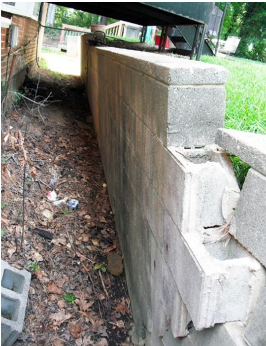
Photo 6. This unreinforced concrete block retaining wall has failed. Failure will adversely affect the building.
