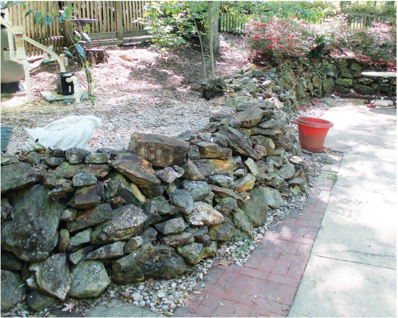
Photo 3. Typical natural stone retaining wall.
