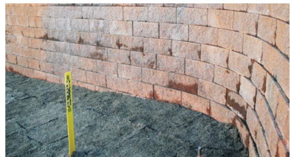
Photo 8. This wall has no visible drainage openings. Water on blocks indicates a possible water management problem.
