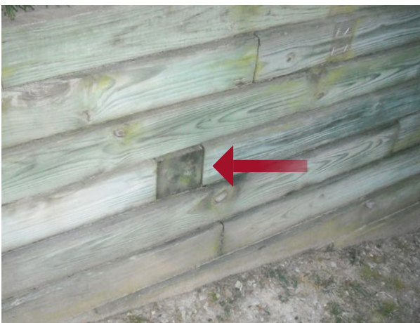
Photo 5. Red arrow points to a tieback.
