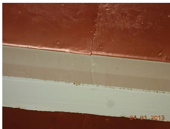
Condensation showing drips at ceiling caused from high humidity, lack of ventilation. The humidity level inside was higher than outside.
