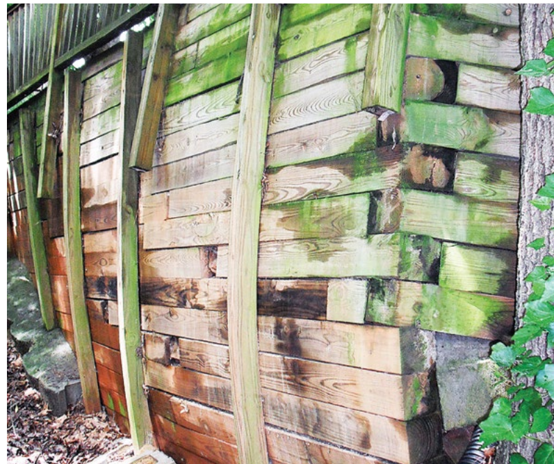
Photo 2. Retaining wall near failure.
