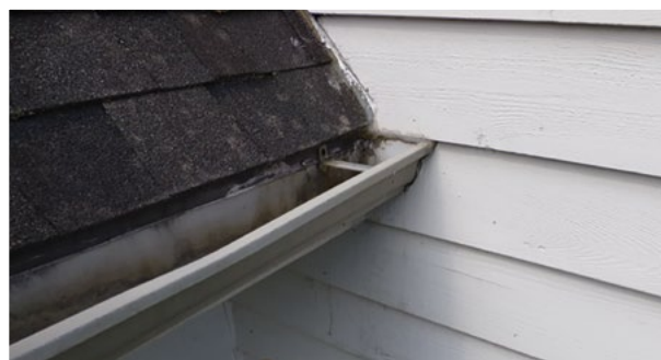
Photo 3. Missing kickout flashing.
