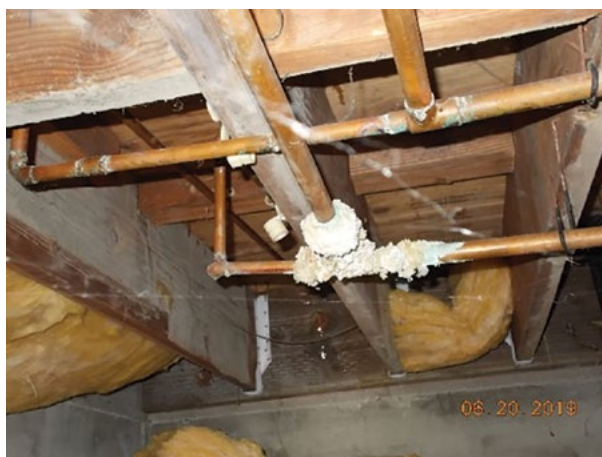
Plumbing supply leak. Excessive corrosion and an active leak. Loose and missing insulation indicates that this may have been a known condition in the past.
