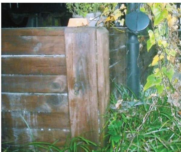
Photo 4. Wood retaining wall with a lateral load. Wood may not be ground contact rated.
