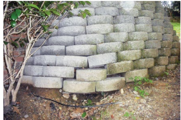
Photo 7. This interlocking block retaining wall does not appear to have a footing. Erosion is occurring under the wall. The wall is probably too tall for the material.
