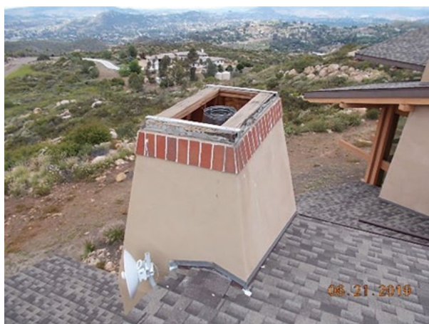
No proper kickout flashing at the roof-chimney edge.
