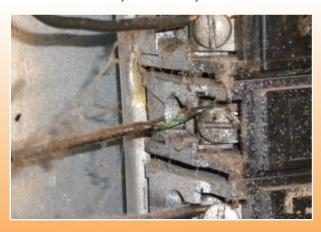
Photo 5. Loose "straight-in" connection on wire-binding screw. This design was only allowed for #10 gauge and smaller per 110.14(A).
