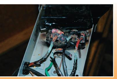
Photo 8. Loose connection at pull-out bar in cheap furnace disconnect.
