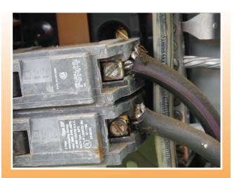
Photo 6. Wires too large for breaker terminals.
