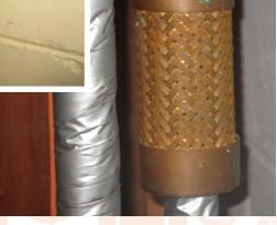
Photo 2. Copper mesh water hammer arrestor.
