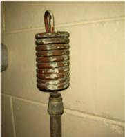
Photo 1. Coil water hammer arrestor.
