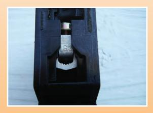
Photo 2. Older GE breaker designed for two wires.
