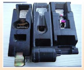
Photo 1. Left to right: Square D breaker designed for two wires, Eaton/ Cutler Hammer CH breaker designed for two wires and Siemens breaker designed for one wire.
