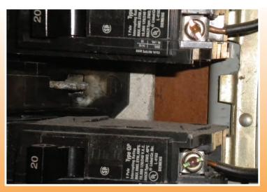
Photo 10. Damaged bus stab.
