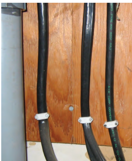
Copper-clad aluminum NM wire (photo credit: Roger Hankey).
