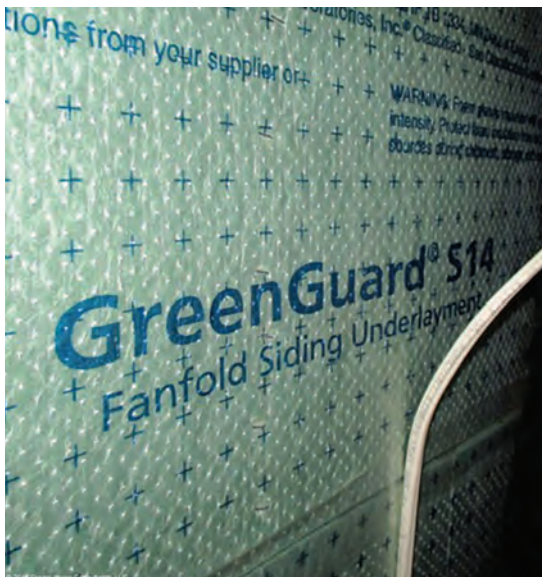
Photo 6. Foam underlayment exposed in attic; warning on label says not to leave exposed.
