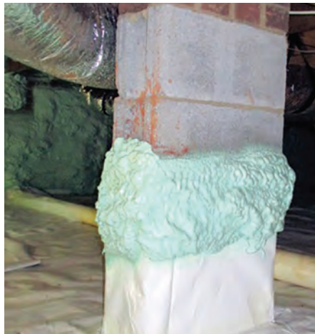
Photo 1. Vapor retarder turned up pier and sealed.
