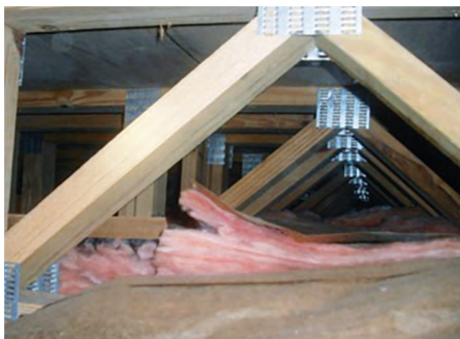
Photo 4. Insulation not in contact with subfloor above floor trusses.
