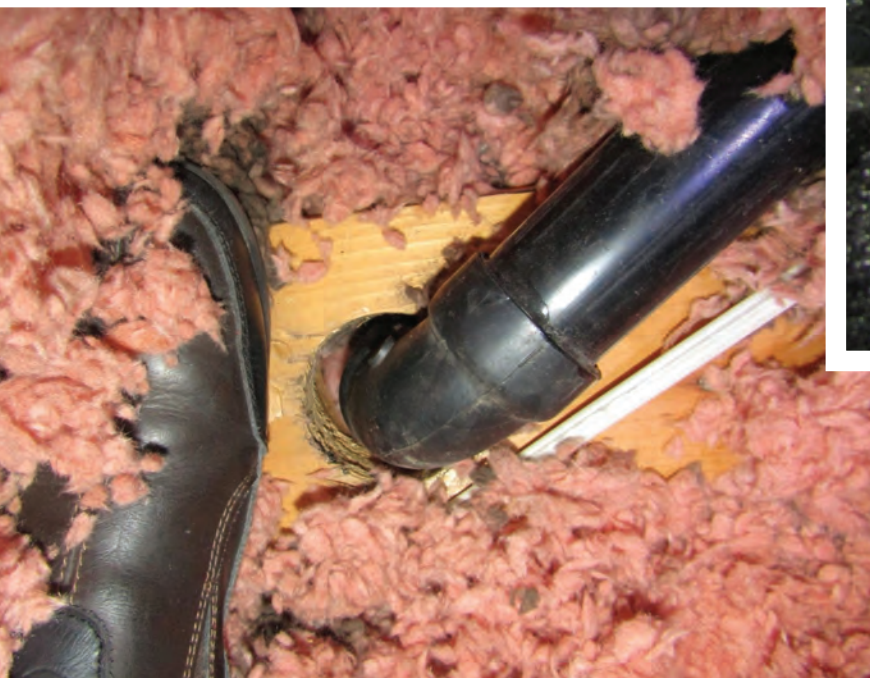
Attic bypass at plumbing vent.
