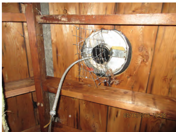
Attic fan with ridge vent.
