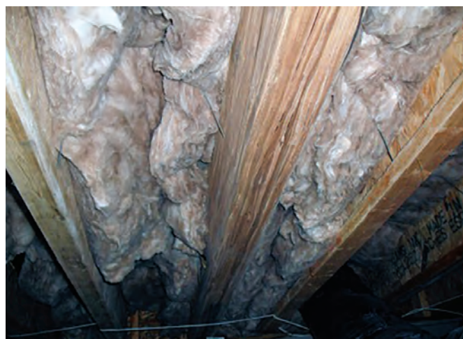
Photo 5. Insulation not cut to fit in space; R-value is minimal.
