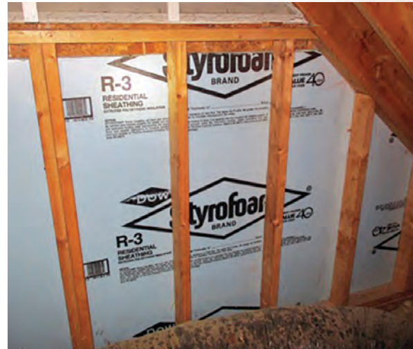
Photo 7. Foam insulation exposed in attic; warning on label says not to leave exposed.
