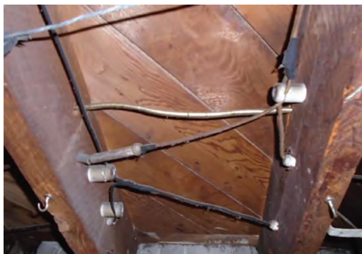
Knob-and-tube wiring
