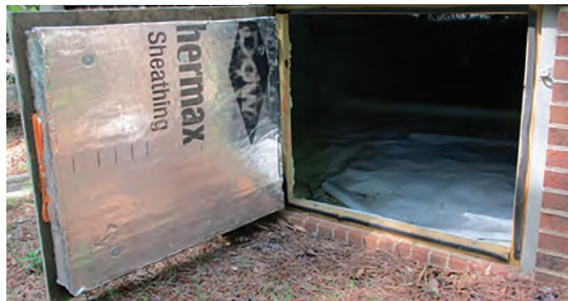
Photo 3. Crawlspace door insulated and weather-stripped.
