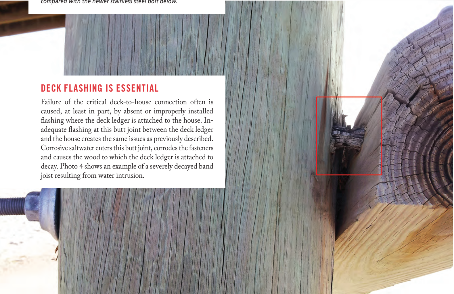
Photo 3. The old bolt is severely corroded and reduced in diameter compared with the newer stainless steel bolt below.
