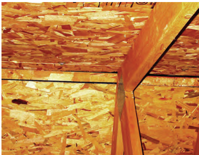
Photo 1. Attic thin strips of OSB.
