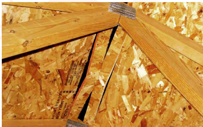
Photo 2. Attic failed OSB at ridge.
